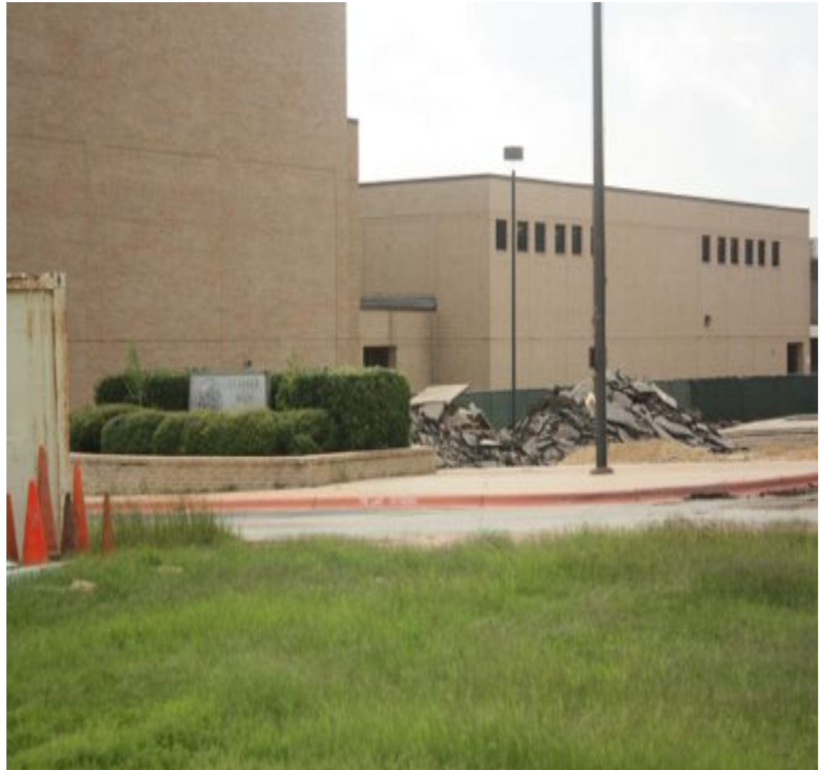
The new building being worked on during school hours.
